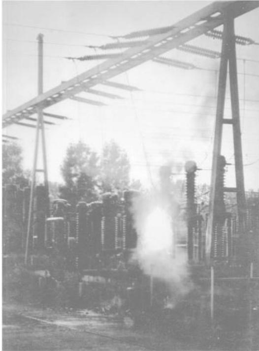
Fig. 2. Standing arc in a substation switchgear
