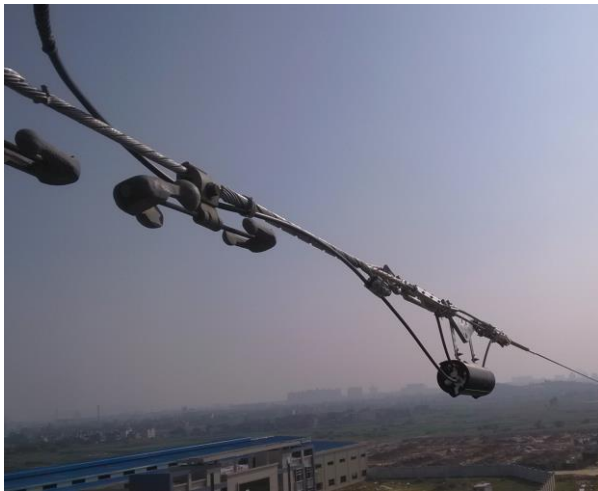
Figure 9. Developed splice tray installed in the field
