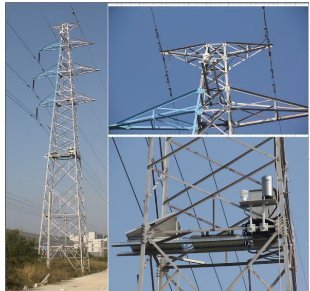
Figure 8. Developed tower terminal unit installed at the tower
